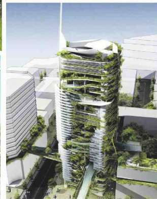
▲ EDITT TOWER In this proposed project in Singapore, heavily planted facades and terraces form a continuous spiral to the top. Total planted area: more than 41,000 square feet, or more than half the building's total area.
